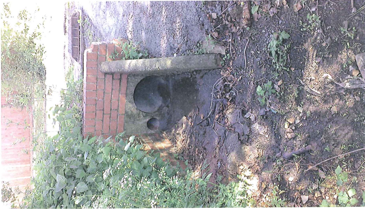
Photo C: Culvert exit from Dyers Road
