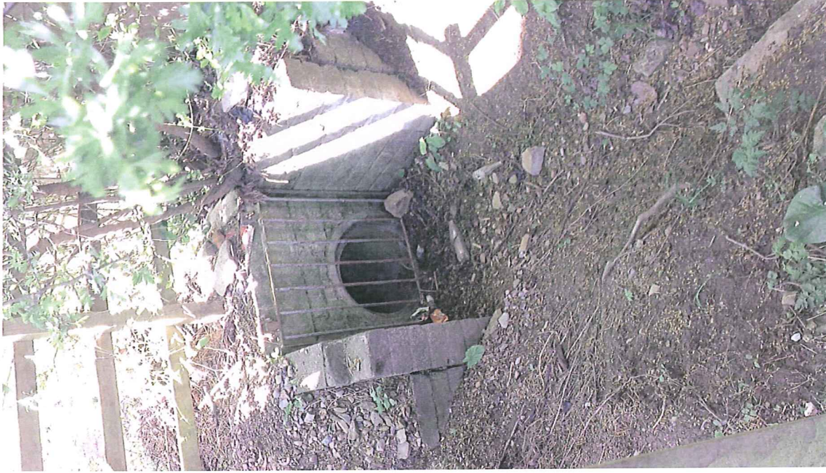
Photo D: Culvert immediately downstream of the site.
